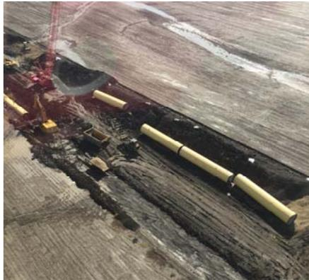
Work in progress on the IPL. Crews laying the 108 inch steel pipes.
