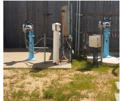
*Rate of flow control actuators*
